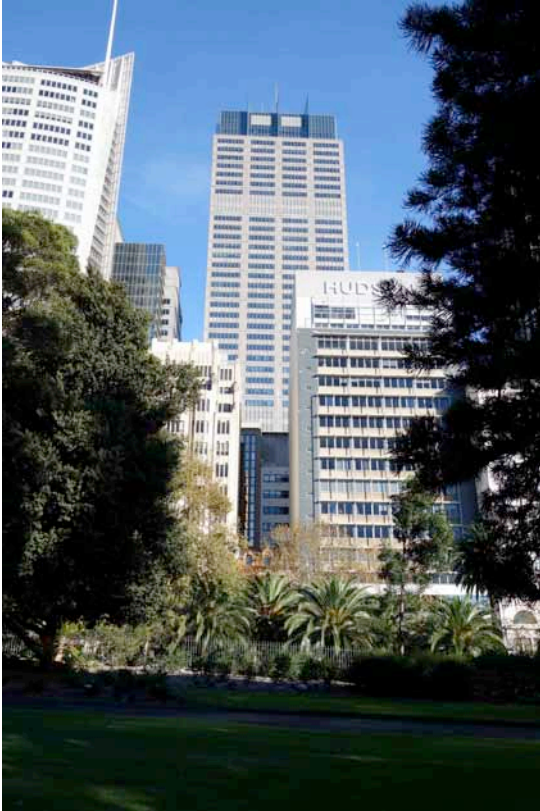
FIGURE 2.13: View E: the attic and roof levels are visible in direct views looking west from a crest on the western side of the Botanical Gardens
