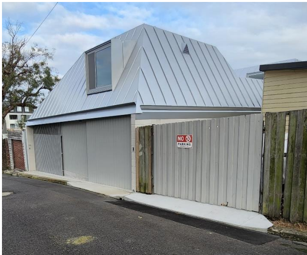
Figure 3 The seamed metal roof in Arcadia Lane.
