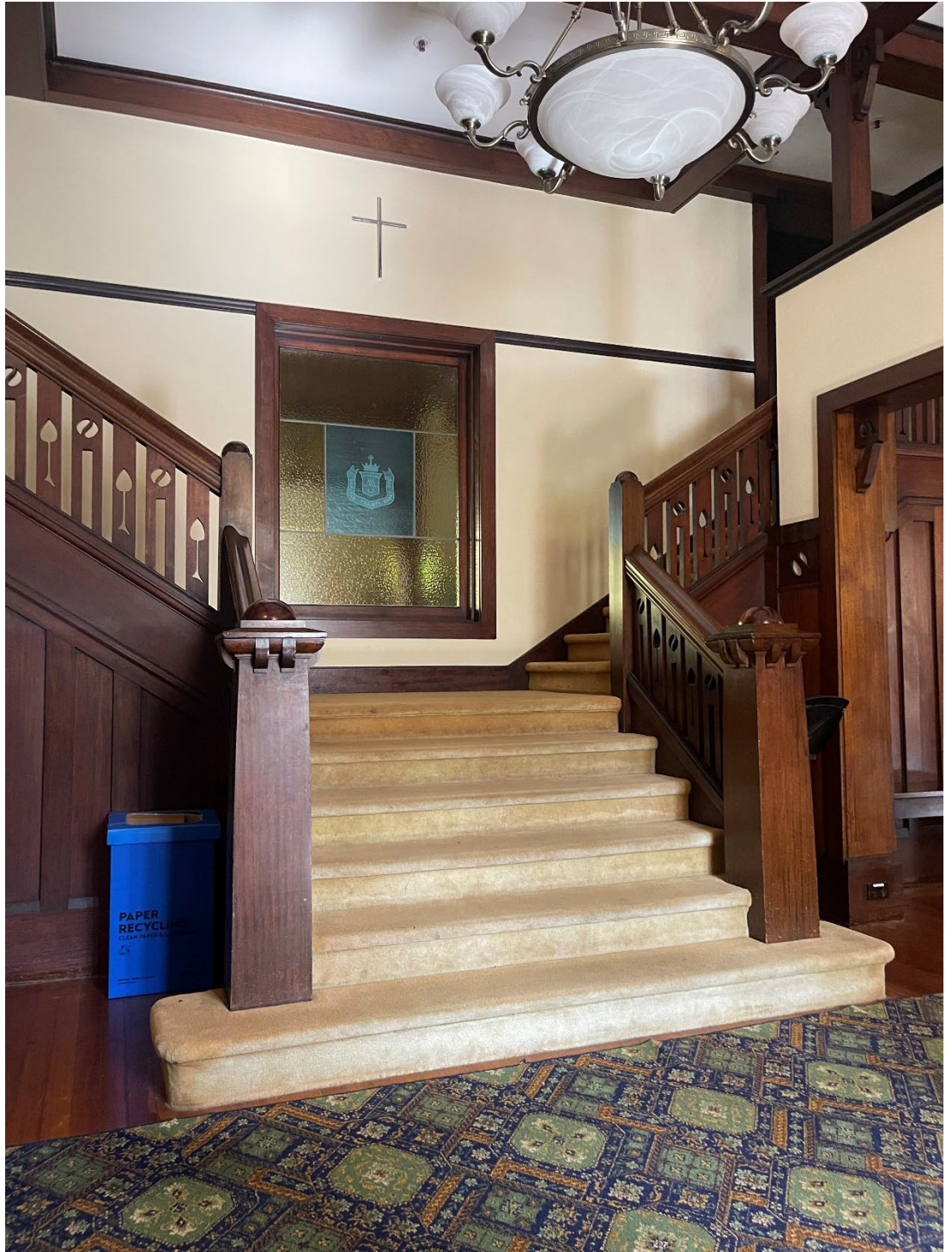
Figure 26: Superior quality joinery, the main entry stairs in Garcia to be retained.
