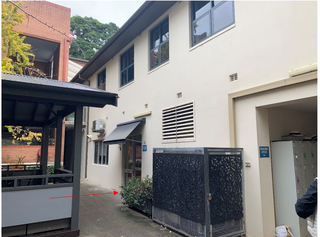
Figure 37: Section of Aikenhead House (constructed 1992) to be demolished to improve external spaces.
