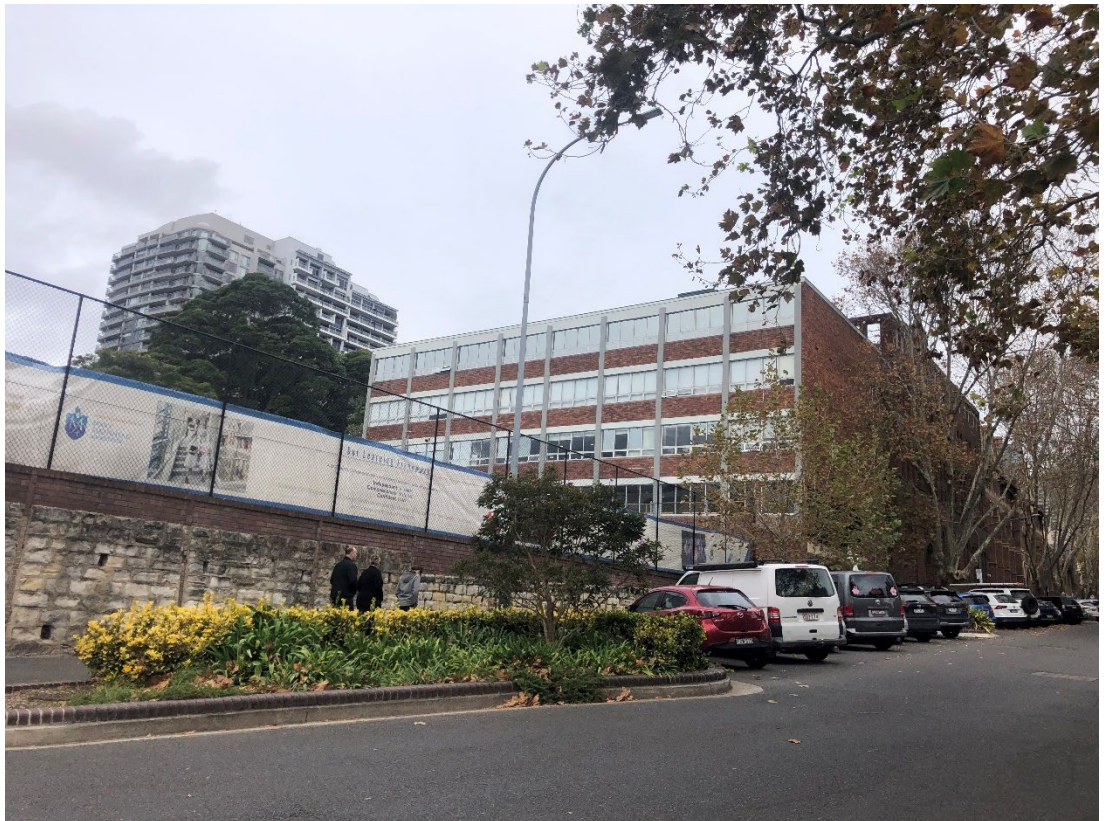
Figure 38: North elevation Vincentia (Low significance). Proposed alterations internally and externally to connect proposed building.
