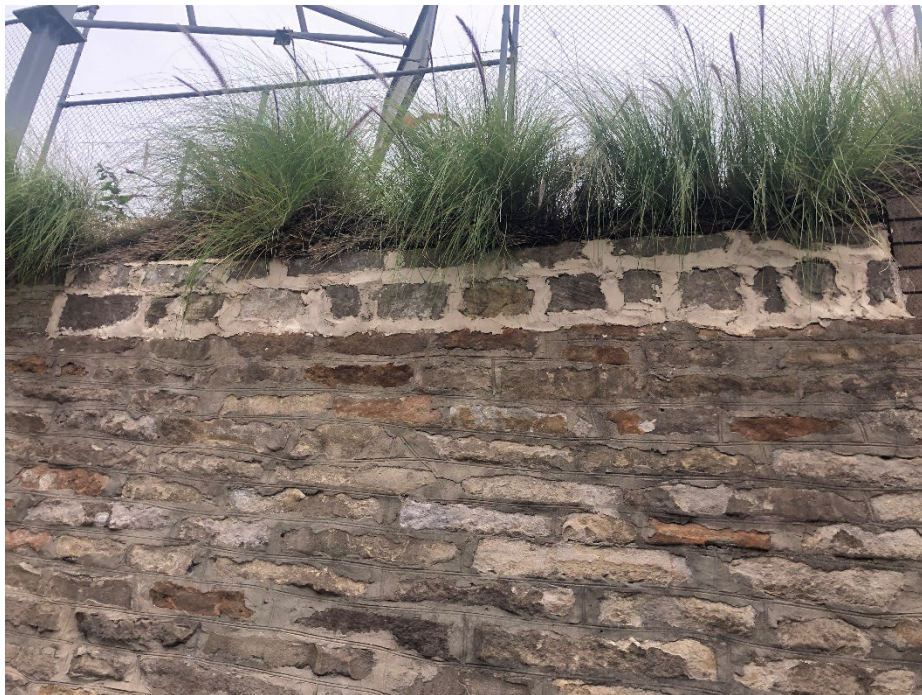
Figure 40: Another area where inappropriate pointing is affecting the condition of the sandstone wall along Challis Avenue
