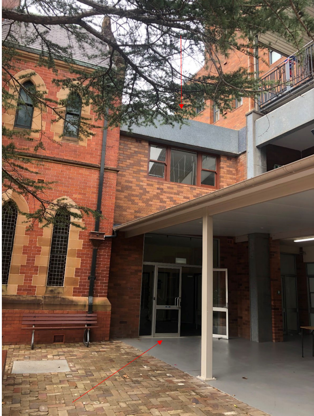
Figure 33: Later addition adjoining the south elevation of the chapel. Internal changes/demolition to this addition are proposed.
