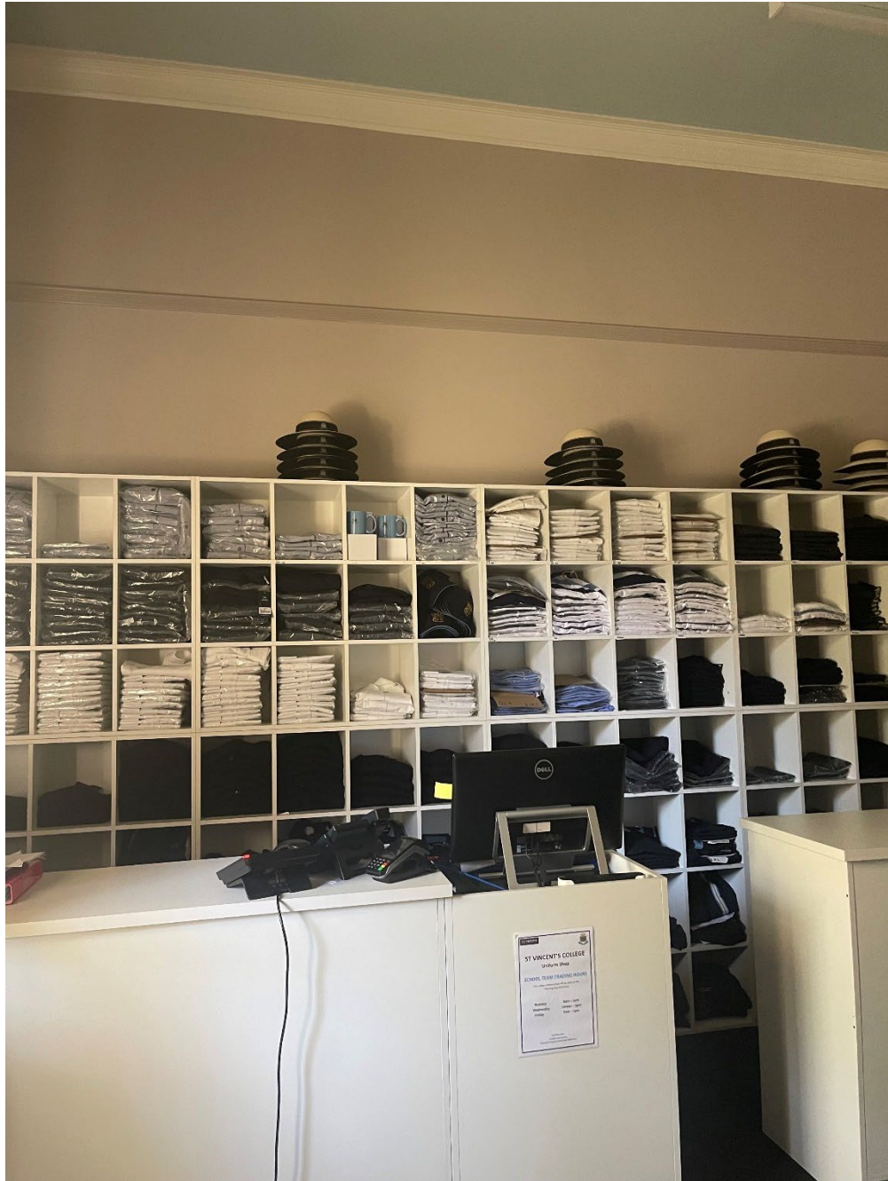
Figure 19: Other side of the wall being removed on Level 3 Garcia which is a later altered element.
