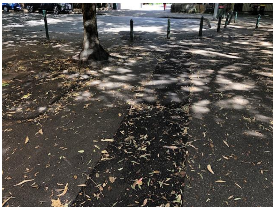
Plate 4: Image showing new trenching below Tree 3. P.Vezgoff
