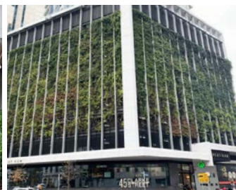
Pre-Grown Green Facades This system provides great foliage cover at installation, instead of waiting up to 2-3 years for coverage.
