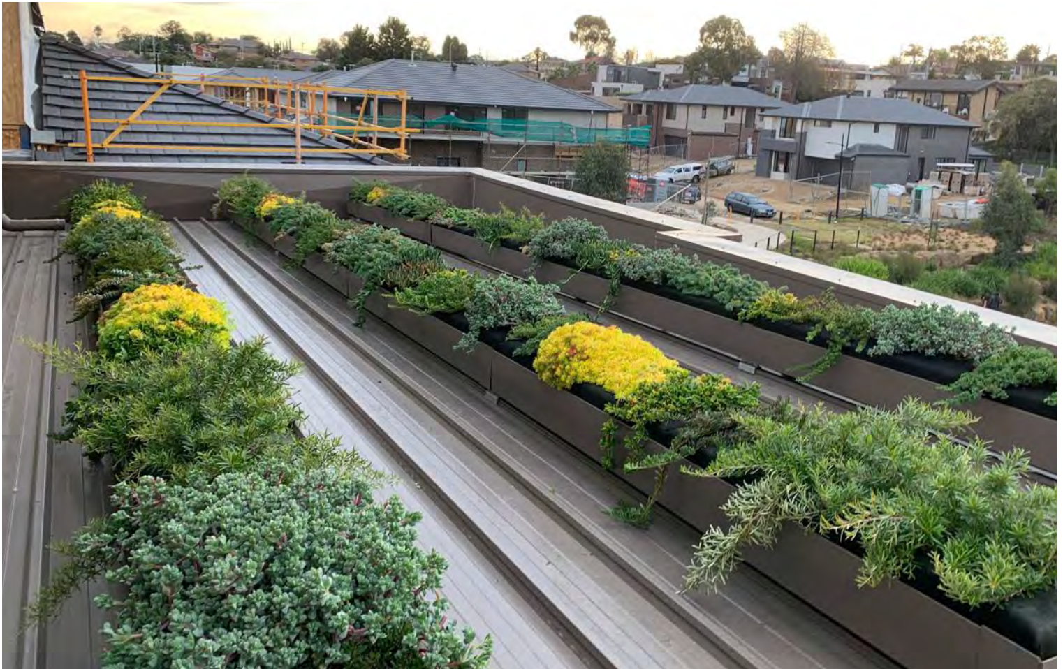
FytoArbour roof garden growth at time of installation
